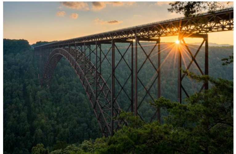
New River Gorge Bridge, West Virginia.jpg
